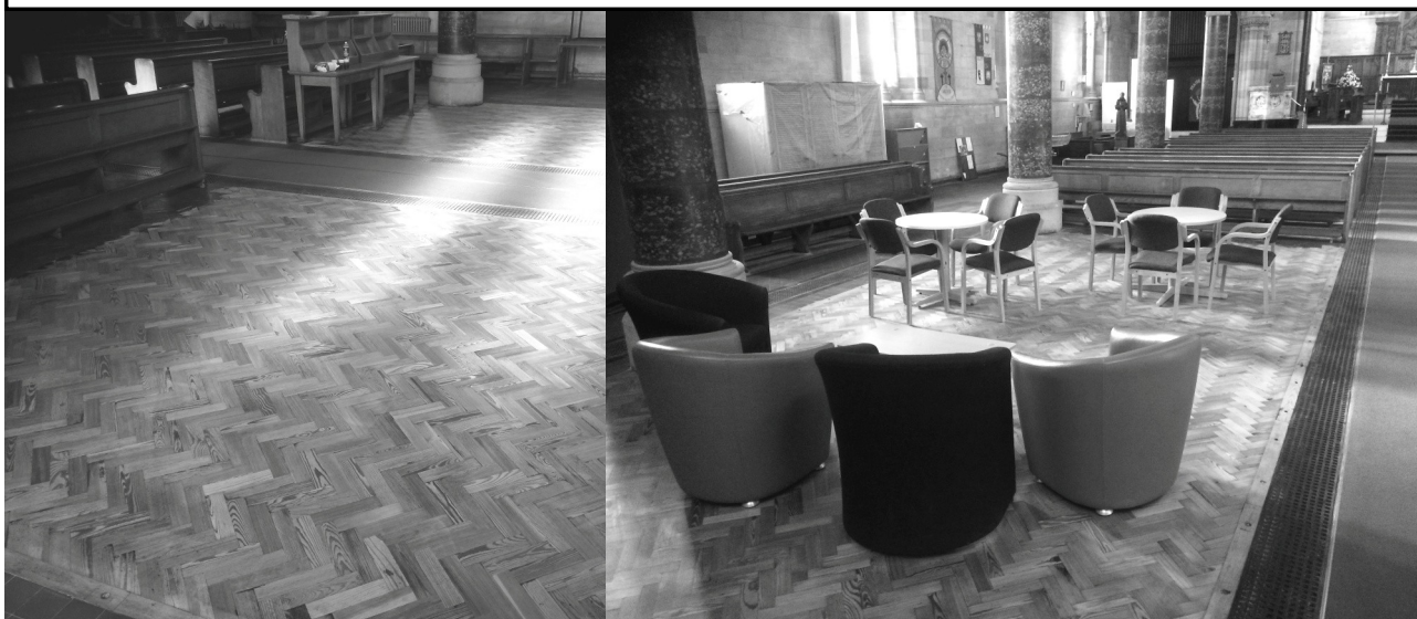
Floor restoration at St Paul's. ABOVE LEFT: just before work began - decades of grime await the attention of the sanding machine. ABOVE RIGHT: the first of several passes with the sander, but the floor is already starting to reveal its true colour. Note the stripes where the pews used to be! BELOW LEFT: the finished floor is left to dry, and is already reflecting the evening sunshine, and making the church feel brighter. BELOW RIGHT: furniture back in place, but still plenty of clearing up to do.
