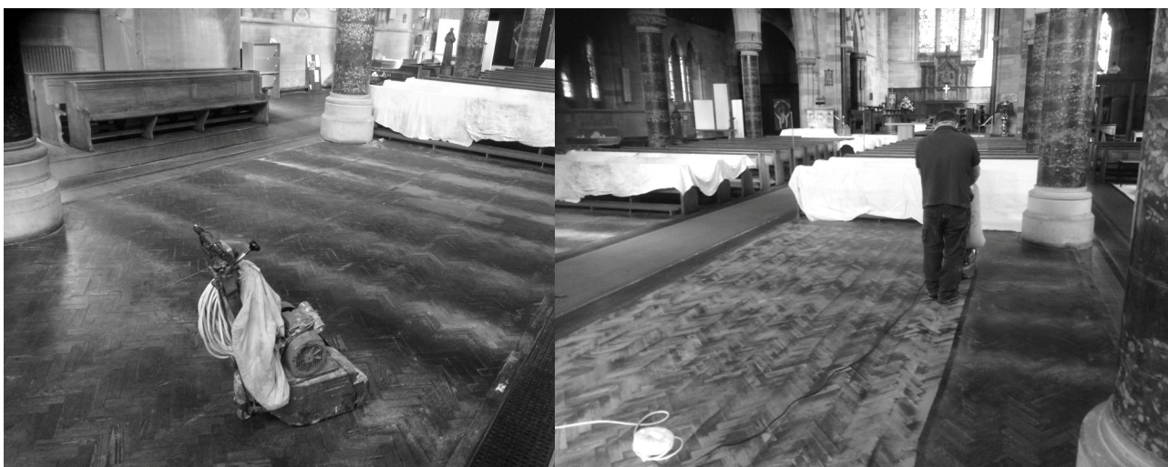
Floor restoration at St Paul's. ABOVE LEFT: just before work began - decades of grime await the attention of the sanding machine. ABOVE RIGHT: the first of several passes with the sander, but the floor is already starting to reveal its true colour. Note the stripes where the pews used to be! BELOW LEFT: the finished floor is left to dry, and is already reflecting the evening sunshine, and making the church feel brighter. BELOW RIGHT: furniture back in place, but still plenty of clearing up to do.
